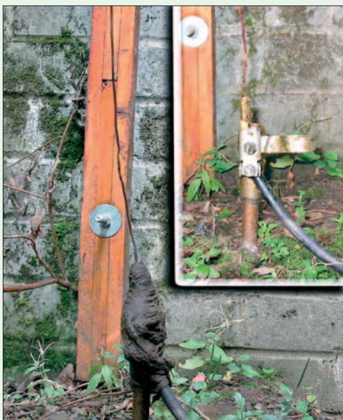
● Fig. 2: After the trimming adjustments, the bottom of the antenna is covered in a thick covering to waterproof the join. The join itself and the 'Tenby' clip are seen in the inset photograph.
